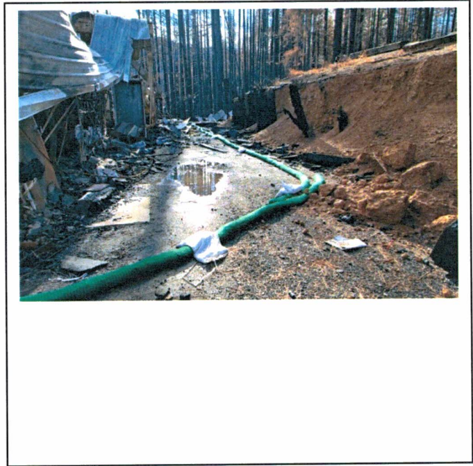
Looking South at Remains of Timber Retaining Wall on Right
